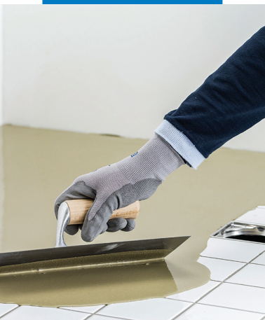
Application of Planex HR with a metal trowel
